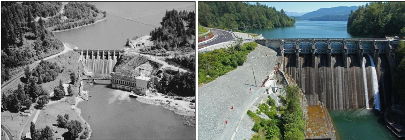
Figure 2: Photos of Ruskin Dam and generating station in 1950 (left) and after the right abutment upgrades in 2010 (right)
